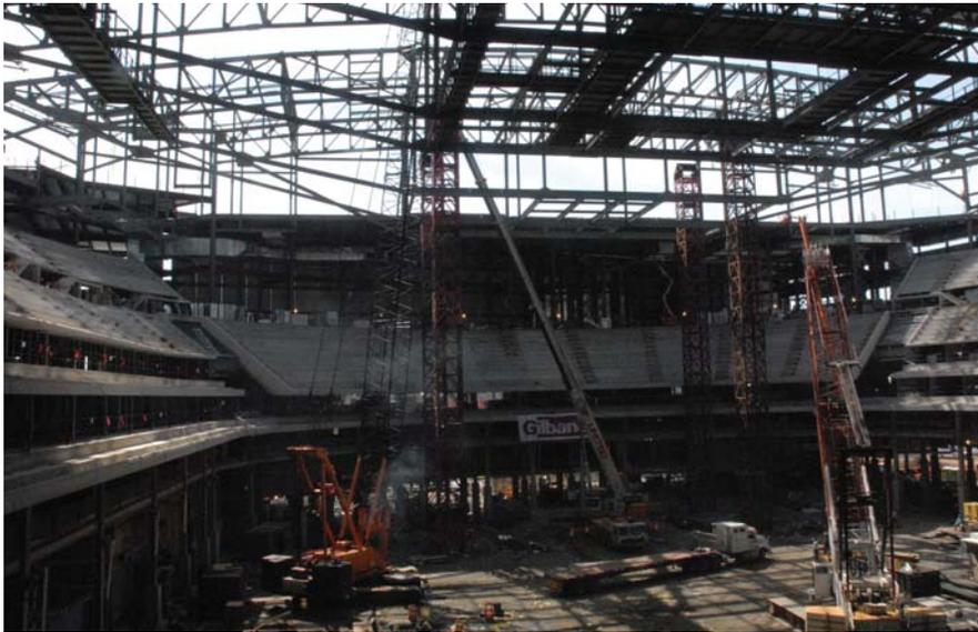
Erecting the roof structure was a major task, requiring shoring towers that needed their own footings. Work progressed on the seating bowl, exterior, and other features while the roof was completed this year.
